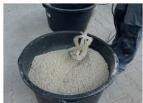
Carefully mix for 3 minutes in an agitator. For an improved mixing result, transfer into a second mortar bucket and re-mix for one minute.
