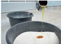
Add the entire contents of the granulate sack into a mortar bucket and add the entire tin of PU binder.
