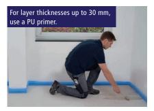
Lay out the edge insulation strips, carefully clean the subsurface and prime for sufficient adhesion with the deep primer.
