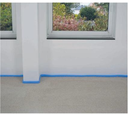
After 3-4 hours' drying time, the surface can be walked on, and after 24 hours, it can be laid. Observe: CompactFloor THERM PU is not a finished usable layer on which floor coverings can be directly laid.
