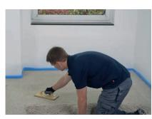
Then smooth the surface with a trowel. The processing time is 30 - 45 minutes.
