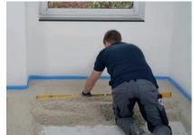
Strip the surface, retaining the height profile.
