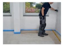
Form dams based on the metre level in the height profile. Layer thickness at least 10 mm to max. 100 mm.
